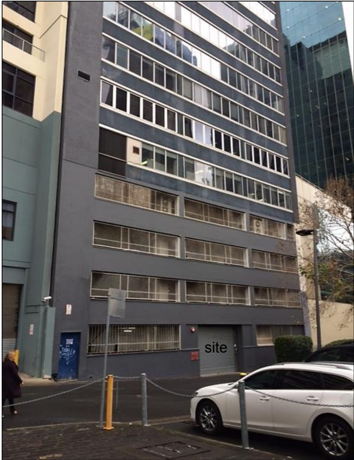
Figure 7: View of site from Jenkins Street
